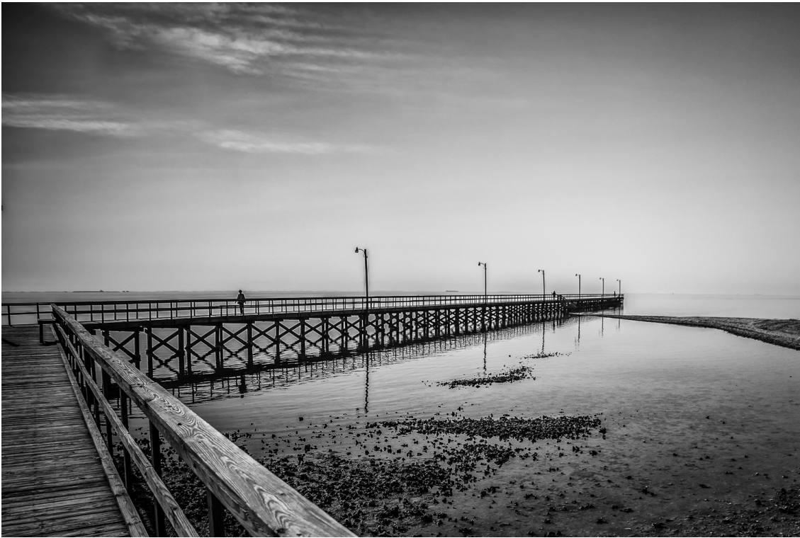
Rockport Beach Pier
